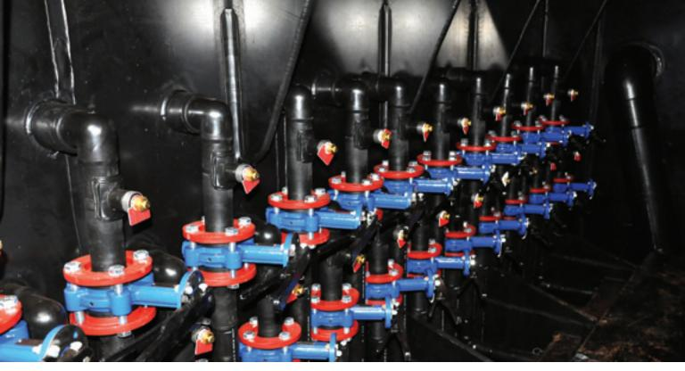
Inside the massive vault, connections are made to bring the boreholes together into a manifold system to take the piping to the ClimaCool® units.
